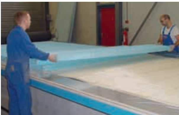
Fig. 07 >> Placing the STYROFOAM™ boards
