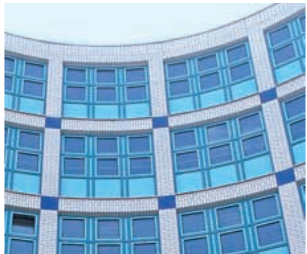
Fig. 21 » ... and spandrel panels
